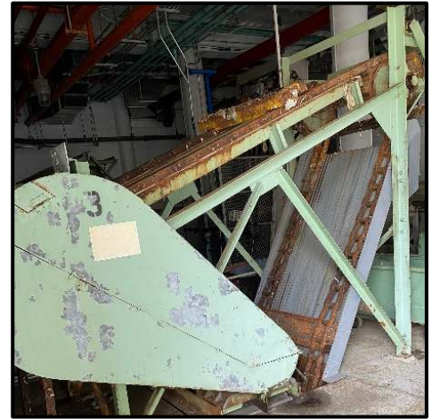
PBU 1 & 2 Installed and in service.
